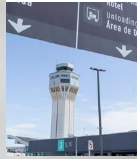
SAN JUAN AIRPORT
